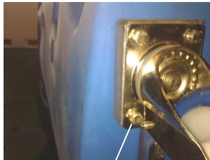
M8 fasteners for assembling the swivel castors
